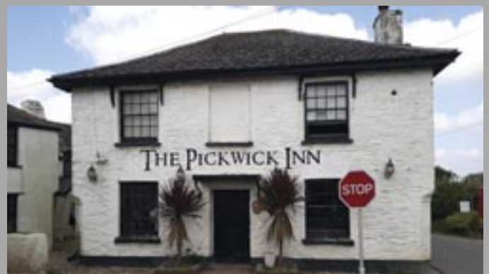
EXAMPLES OF LISTED BUILDINGS
