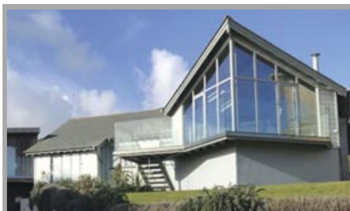
• MODERN EXTENSIONS TO HOUSE AT BIGBURY ON SEA
