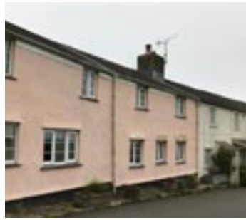
2 - 1 and 2 Court Cottages, Bigbury Village
